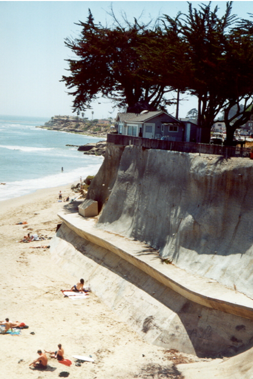
Photo 8. Private residence armoring and seawall, west of Larch Lane.
