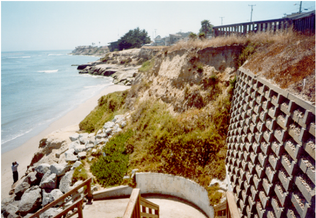
Photo 10. Stairs and crib wall (retaining wall) at 38 th Avenue.
