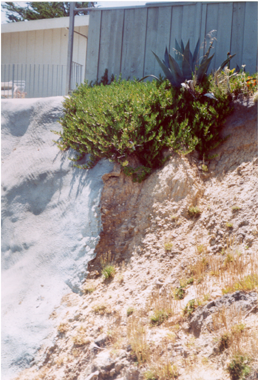
Photo 16. Armoring (private residence) against exposed cliff face, near 41 st Avenue.
