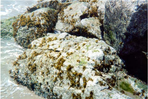
Photo 30. Algae on existing rock riprap. Looking upcoast from stairs near Larch Lane.
