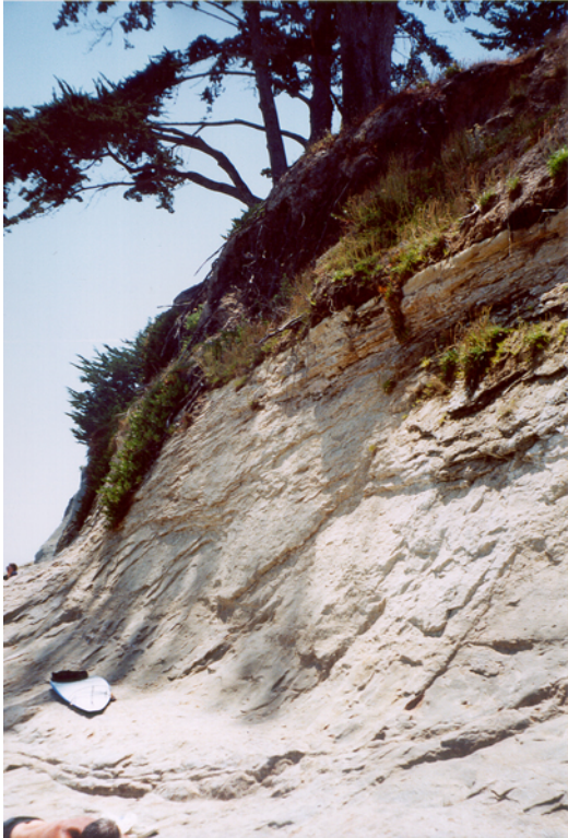
Photo 22. Thick Purisima formation with vegetation covering terrace.
