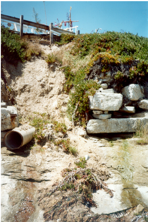
Photo 12. Drainage below East Cliff Drive.
