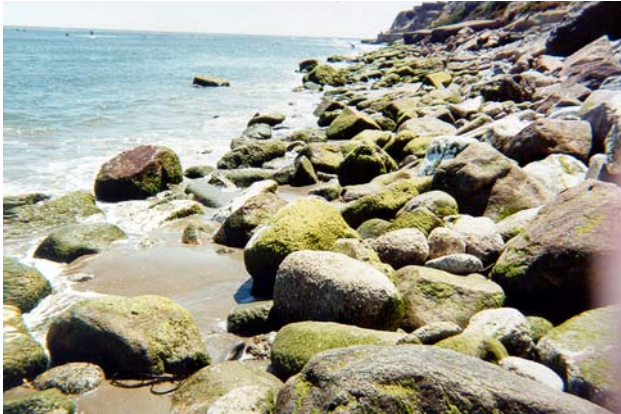
Photo 29. Algae on existing rock riprap. Looking upcoast from stairway and restroom, near 35th Avenue.
