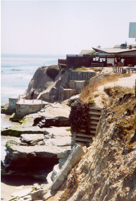
Photo 2. Bluff protection and engineered terraces near Pleasure Point Park.
