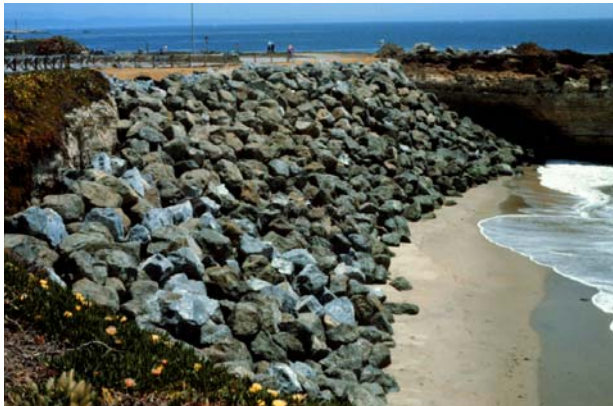
Photo 33. Example of riprap revetment footprint in Central California.
