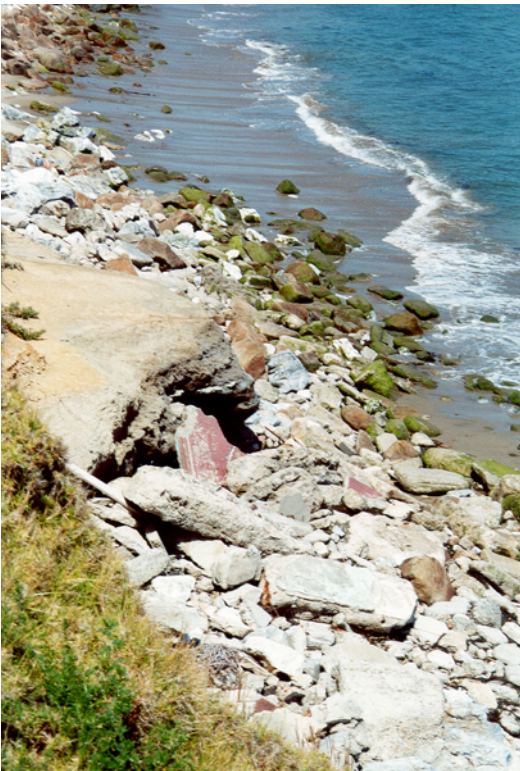
Photo 4. A close-up view of the concrete rubble and rock riprap.
