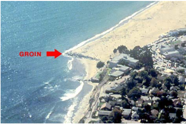
Photo 34. Groin at Capitola Beach.
