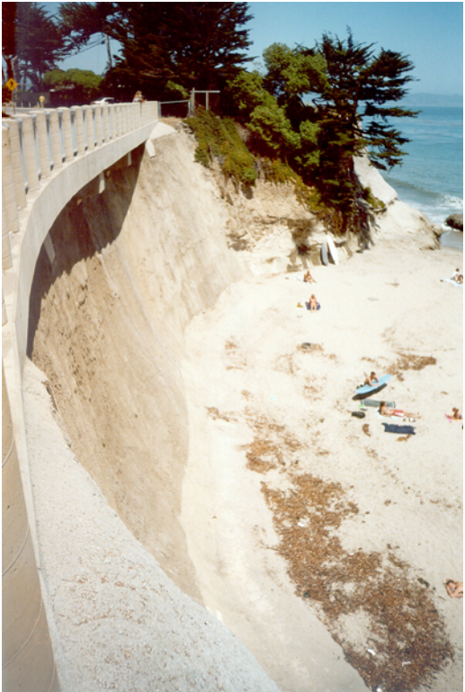
Photo 7. Larch Lane emergency armoring, looking downcoast.
